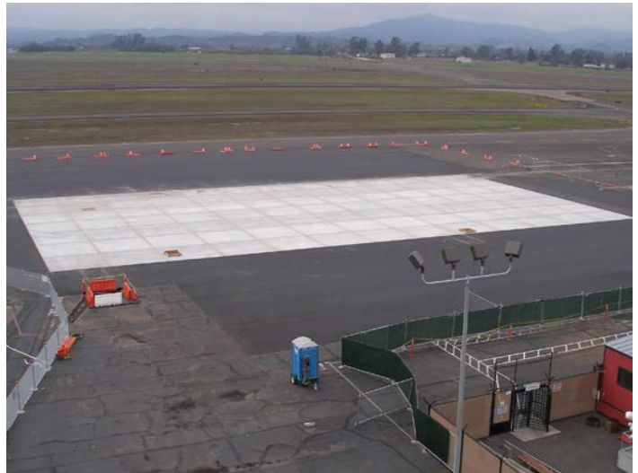
Concrete pad complete.
