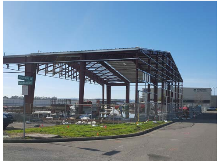
Construction as of January 15, 2016.
