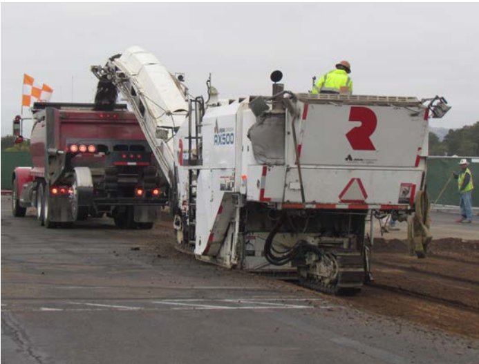
Pavement removal.
