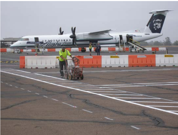
Temporary markings for the new Security Identification Display Area (SIDA) for commercial aircraft positions.
