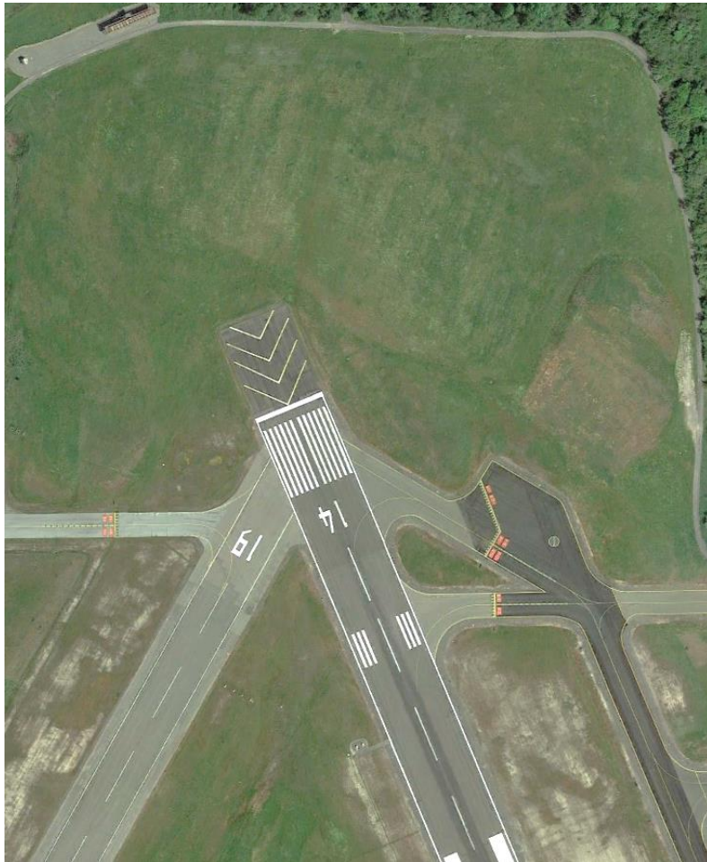
Figure 3-2: Runway 14 & 19 Approach Ends, March 2013
